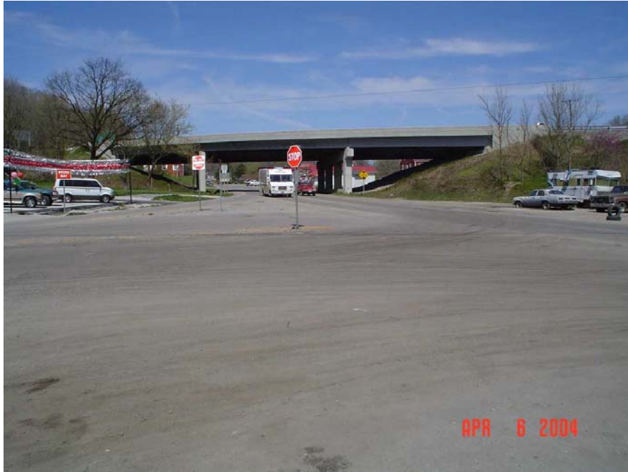
KY 11 INTERSECTION WITH HAL ROGERS PARKWAY OVERPASS IN BACKGROUND
