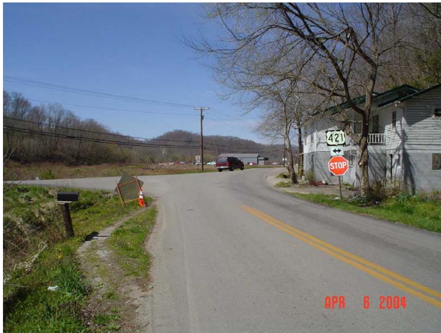
NORTHWEST VIEW OF US 421 AND KY 149 INTERSECTION
