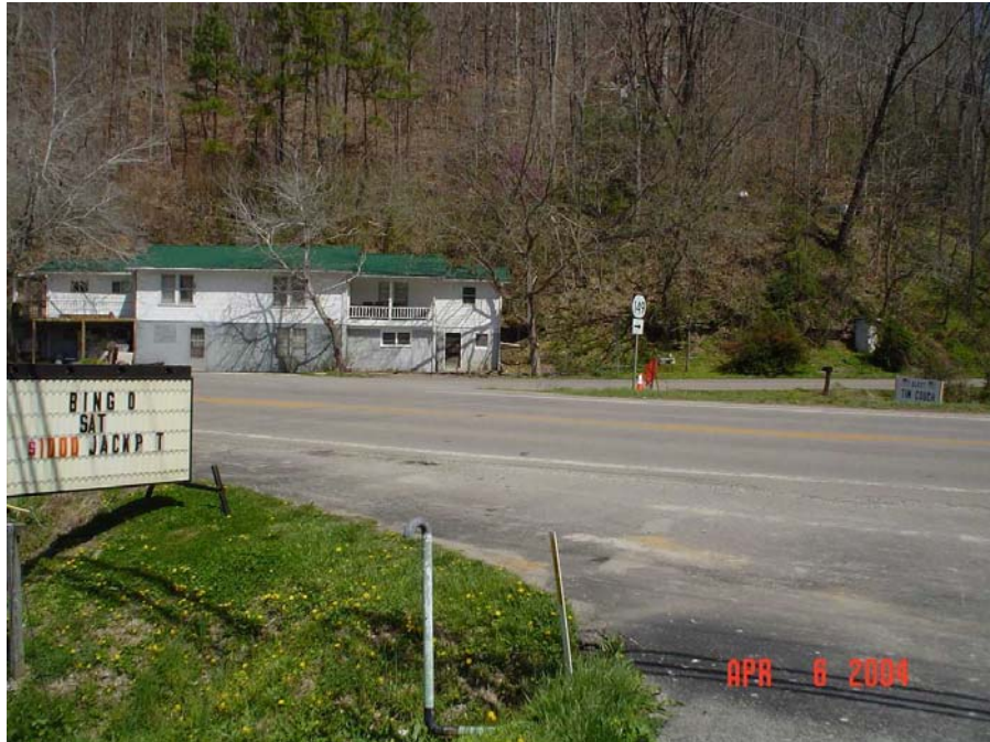
NORTHEAST VIEW OF US 421 AND KY 149 INTERSECTION
